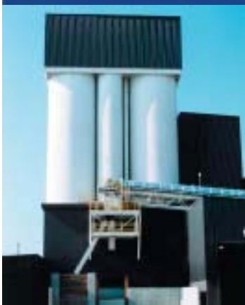
545 metric tonnes/day (600 tons/day) float glass batch plant
