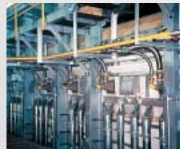
Oxy-fuel furnace melting C-Glass and performing at 250 metric tonnes/day (275 US tons/day) at 850 kcal/kg (3.0 MBTU/US ton)
