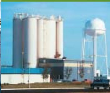
Batch plant for 680 metric tonnes/day (750 US tons/day) production and nominal storage of one (1) week per ingredient
