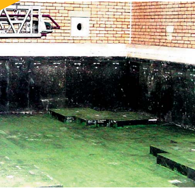
Electric melter built on the "square pattern"
